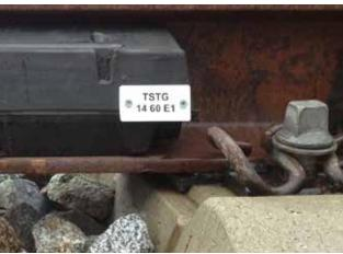
The final position of the fastening clamps is correct (Optional - Depending on rail infrastructure operator) owner) when installation is completed, fix the batch/ job number labels to the absorbers, as required by the client. Typically this will be with self-tapping screws or ,gun'-fired staples.
