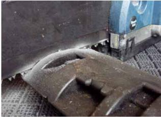
If required, the length of a absorber can be reduced at each end by a strict maximum limit of 30 mm (using a low speed cutting tool - typically a hand saw or powered (reciprocating) equivalent). This may be necessary to accommodate:
