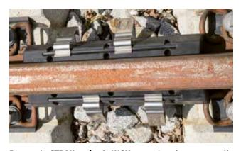
one on each side of the rail, fit two fastening clips into profiled grooves on each absorber, making sure that the clips are evenly spaced and there are clear gaps between all 4 clips before springing them in to place.
