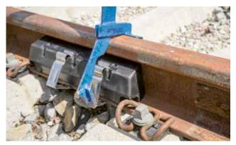
Afterwards, use the installation lever arrested on the Final position of the fastening clamps on the side of rail head and **push** the clamps through under the rail foot and bring them into their final positions. The final position is indicated by a "click" sound.
