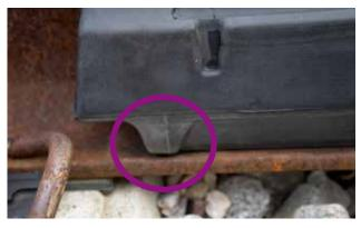
Place the STRAILastic\_A INOX 2.0 absorbers into the When the indicator (see circle) is vertically flush with installation position on the rail profile (normally the rail foot the absorber should be in full contact
