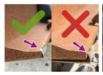
if the two lateral straps on the clamp enclose the rail foot completely.
