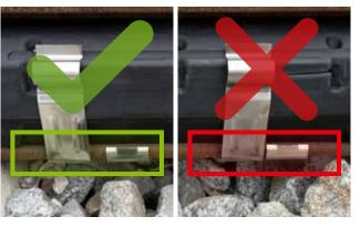
For each STRAILastic\_A INOX 2.0 absorber, normally Important check - the opposing clips must not touch each other!
