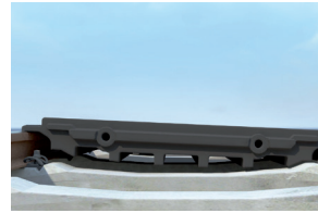
Insert the pedeSTRAIL inner panel on one side with its lip under the rail head and grease the lip on the other side with the assembly paste.
