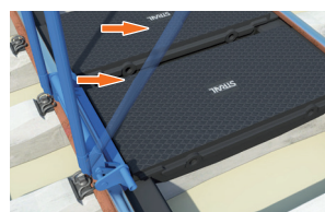
Press the edge of the panel against the installation lever until the lip slides under the rail head.
