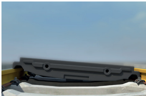
Insert the innoSTRAIL inner panel on one side under the rail head and grease the flange groove support on the other side with the assembly paste.
