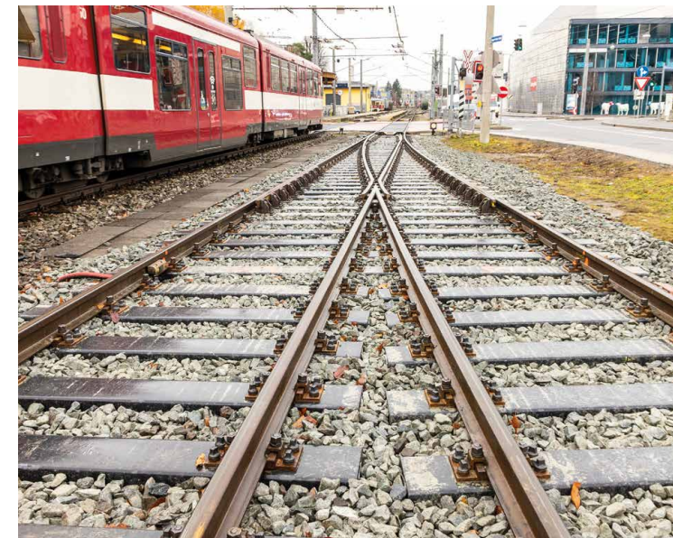
Better screw pull out forces than wood/concrete
